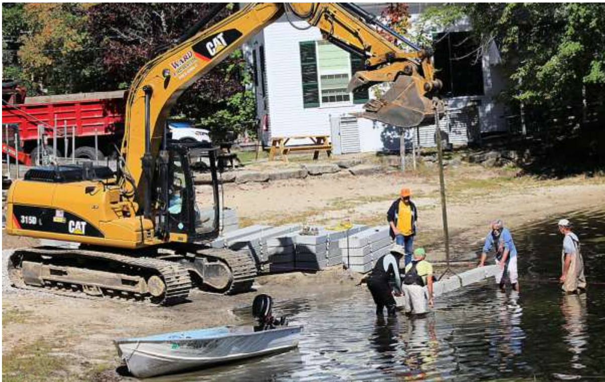
The Keoka Lake boat ramp project began Sept. 13 with the installation of 40 concrete pavers. Jeff Ward made the project possible with his donated time and equipment. The KLA and the town split the project's cost.
