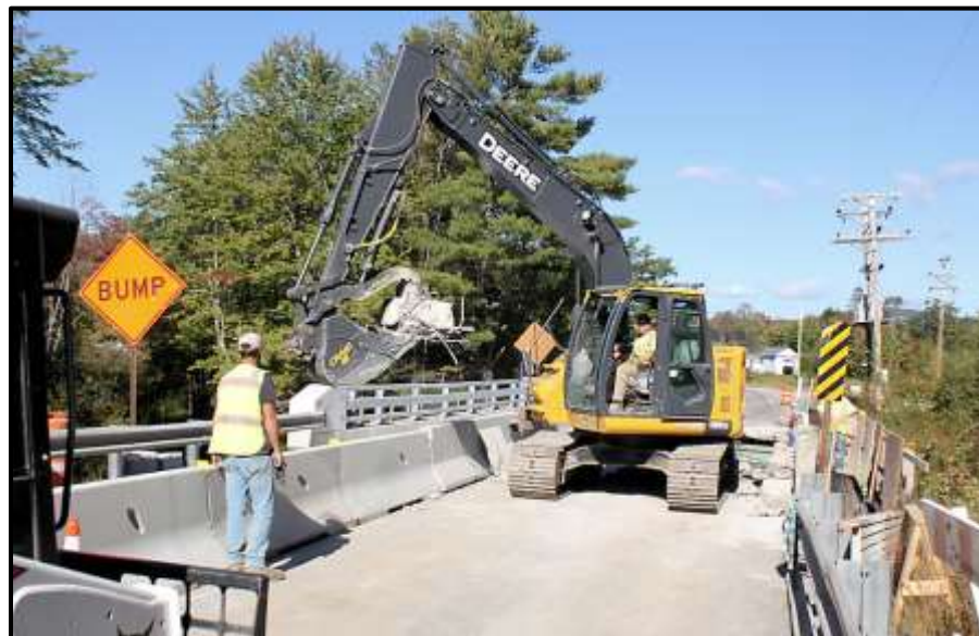
The Horrs Bridge deck replacement on Rt. 35 over Crooked River was completed in late fall. The deck of the 70-year old bridge was widened from 24 to 28 feet.
